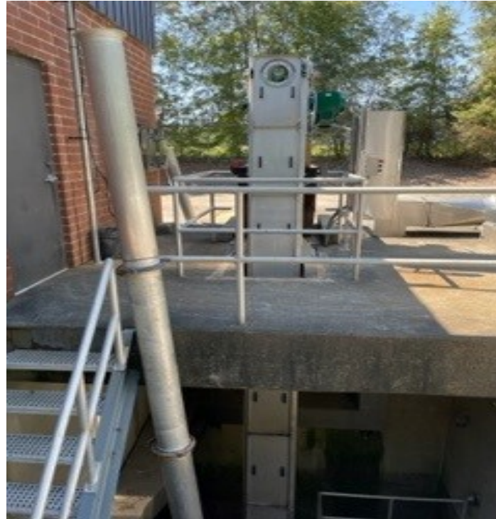
New Hope L/S Bar Screen Replacement $335,400 Completed.
