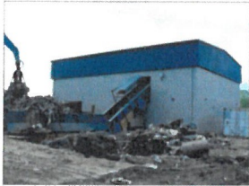
Figure 8: Shredder system enclosure (right side)
