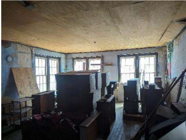
Second Floor storage room
