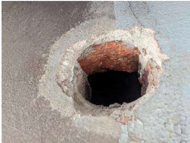
Abandoned Penetrations of Brick Masonry Wall
