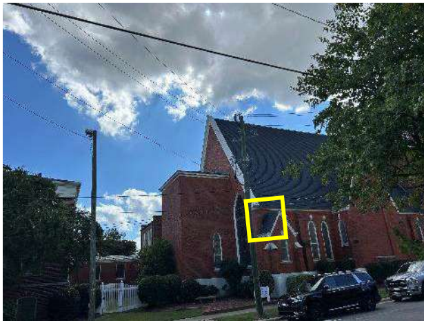
Pilaster Extends Beyond Wall Damming Water at Corner, Internal Gutter is Present
