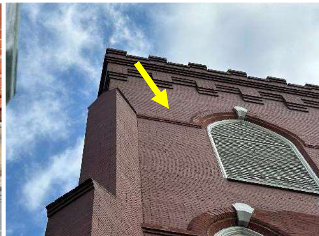
Corbelled Brick Location
