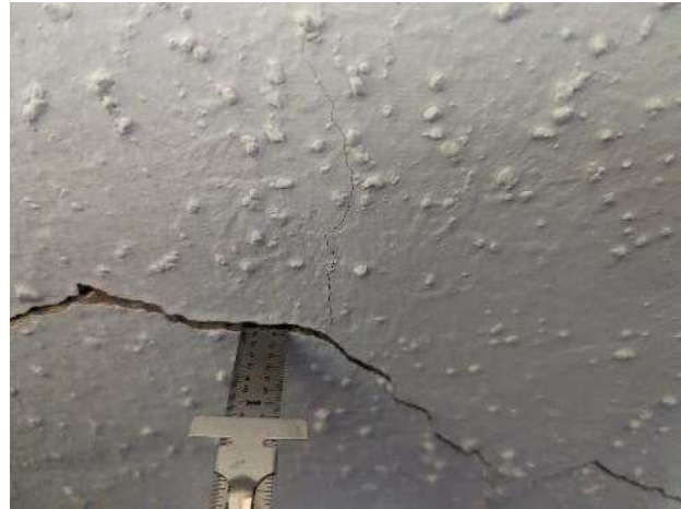
Cracked Plaster Typically Underneath Windows
