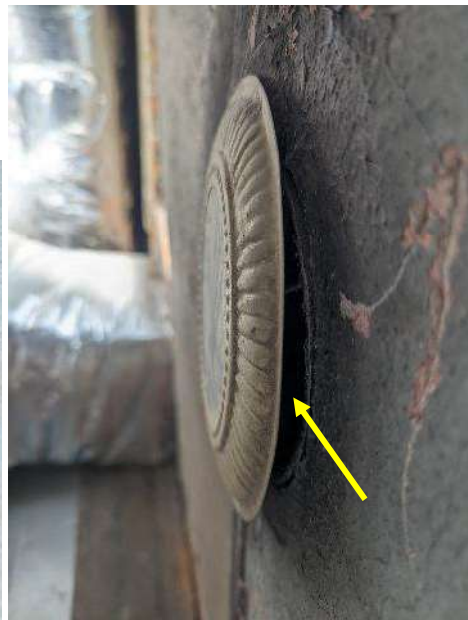
Abandoned Penetrations of Brick Masonry Wall
