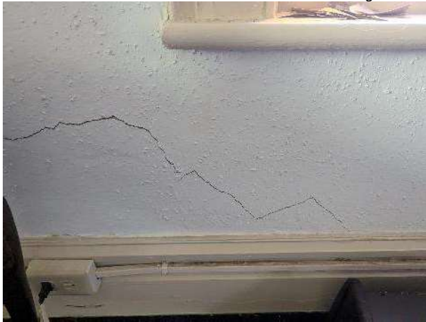
Cracked Plaster Typically Underneath Windows
