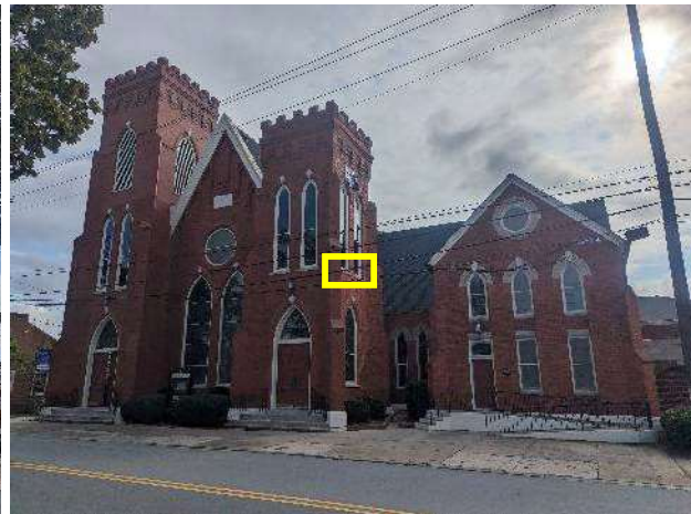
Water Test #02 Location
