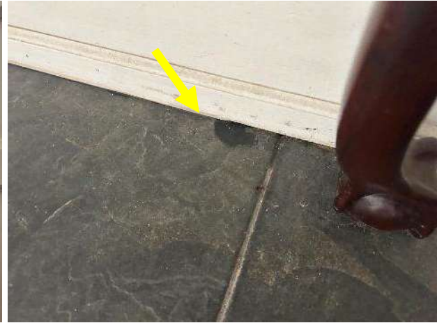
Water Infiltration Noted at Two (2) Locations Below Window Area
