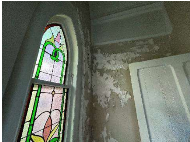
Damaged Plaster/Paint
