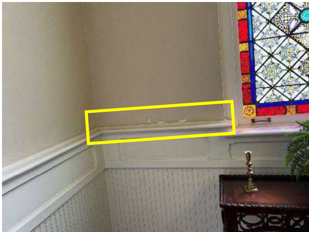
Water Staining/Damage at Paint/Plaster at Transition to Paneling
