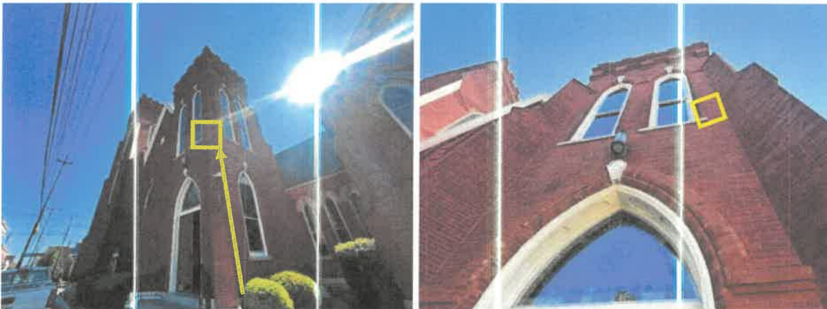
Excavation #01 - Approximate Location at Interior Excavation of South Tower
