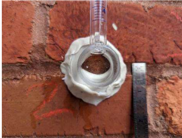
Rilem Test Tube – Bed Joint: Wetting / Absorption of Mortar during Testing
