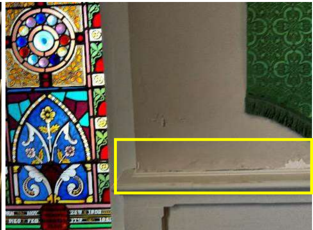
Water Damage at Transition to Paneling
