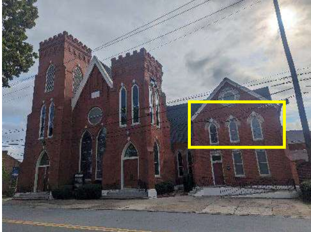
Southern Section of Building
