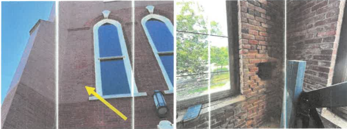
Newer Exterior Pressed Brick Location
