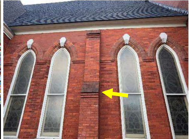
Interior Leakage Centered on Pilaster
