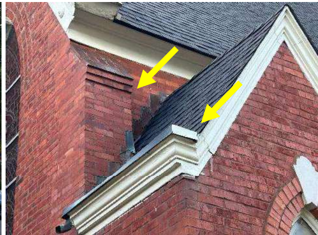
Pilaster Extends Beyond Wall Damming Water at Corner, Internal Gutter is Present
