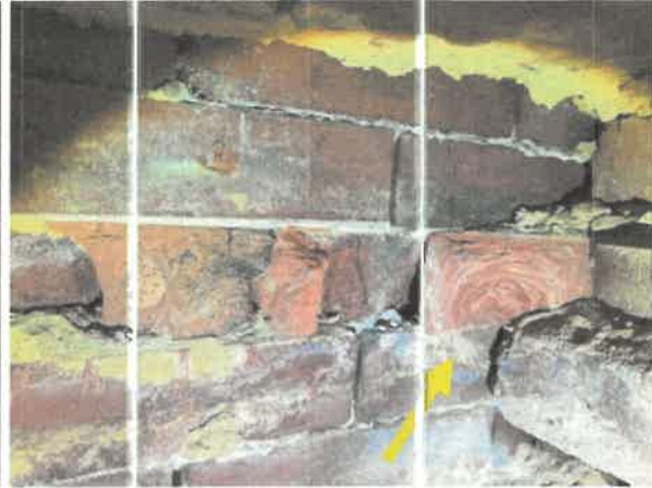
Skewed Header Course Discovered
