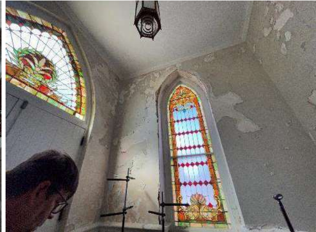
Damaged Paint and Plaster Throughout
