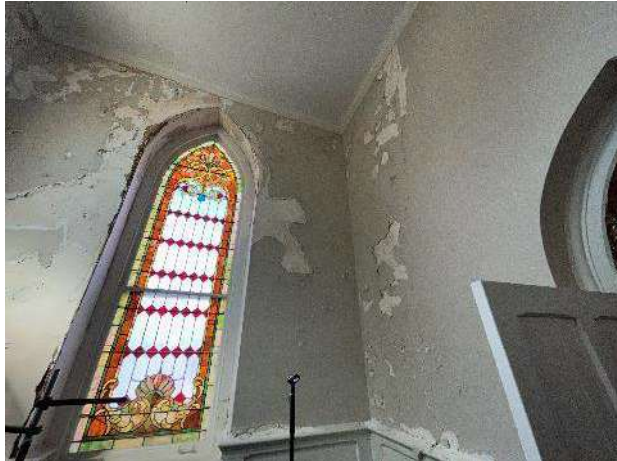
Damaged Paint and Plaster Throughout
