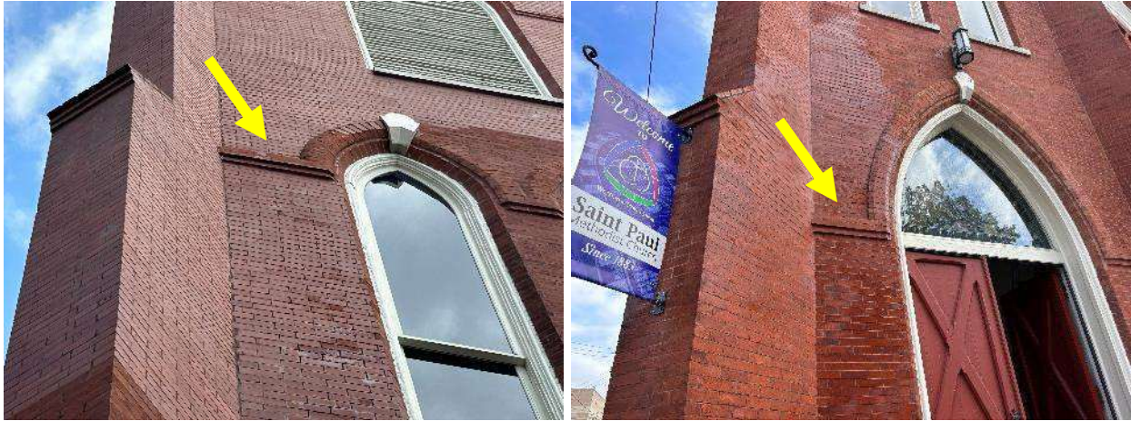
Corbelled Brick Location
