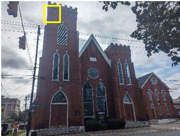
Water Test #01 Location
