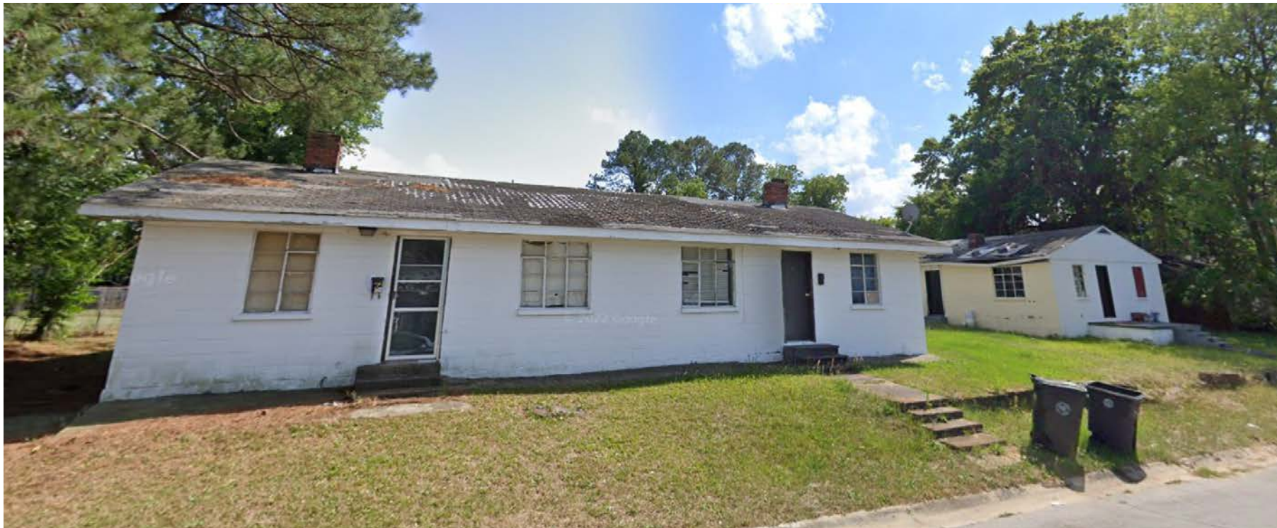
312/314 Existing Building Conditions @ Olivia Lane
