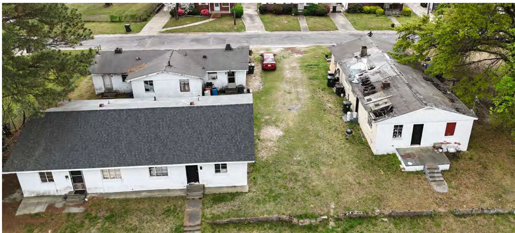
Aerial of Existing Building Conditions @ Olivia Lane
