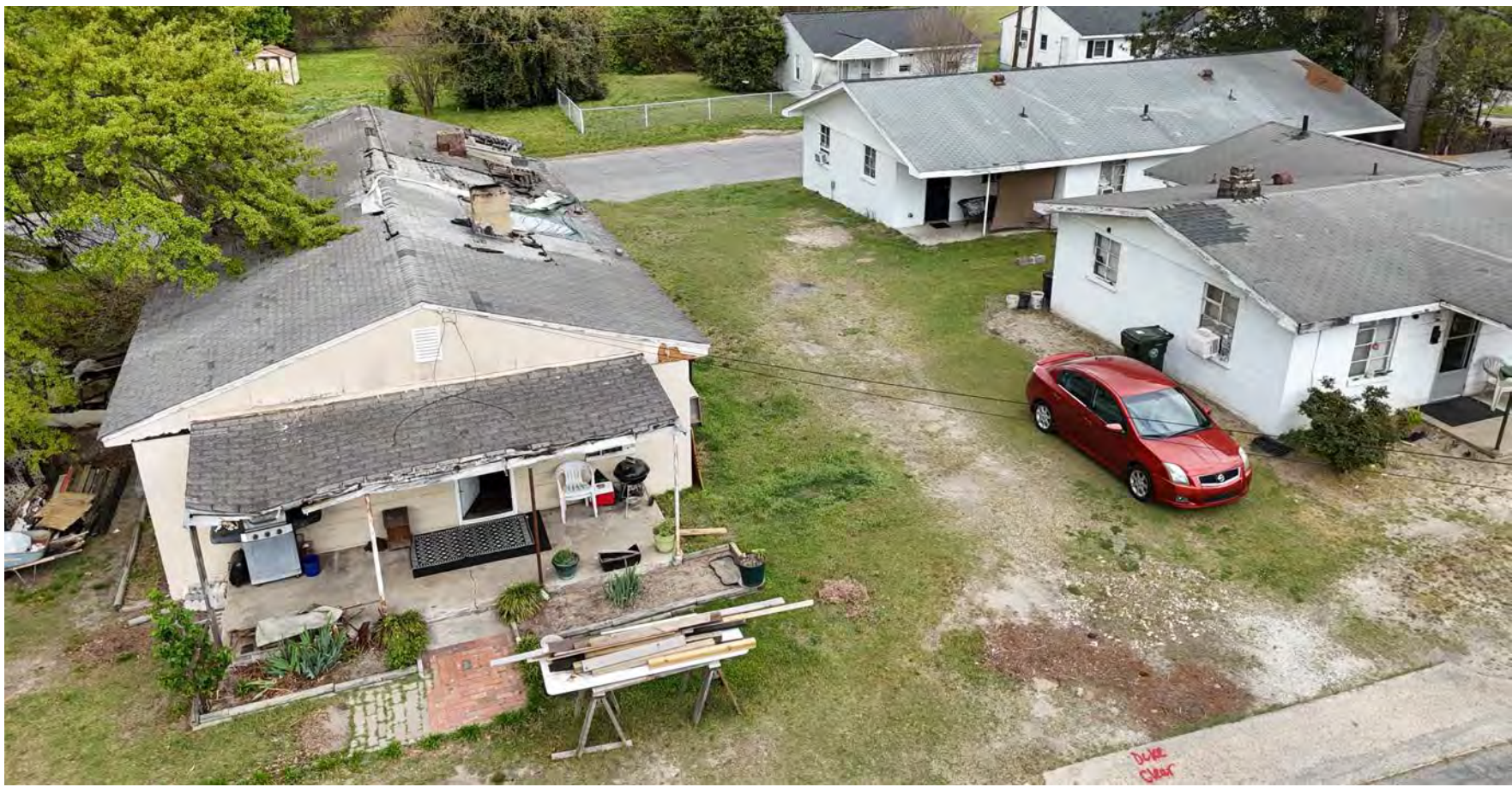
Aerial of Existing Building Conditions @ Wilmington Ave
