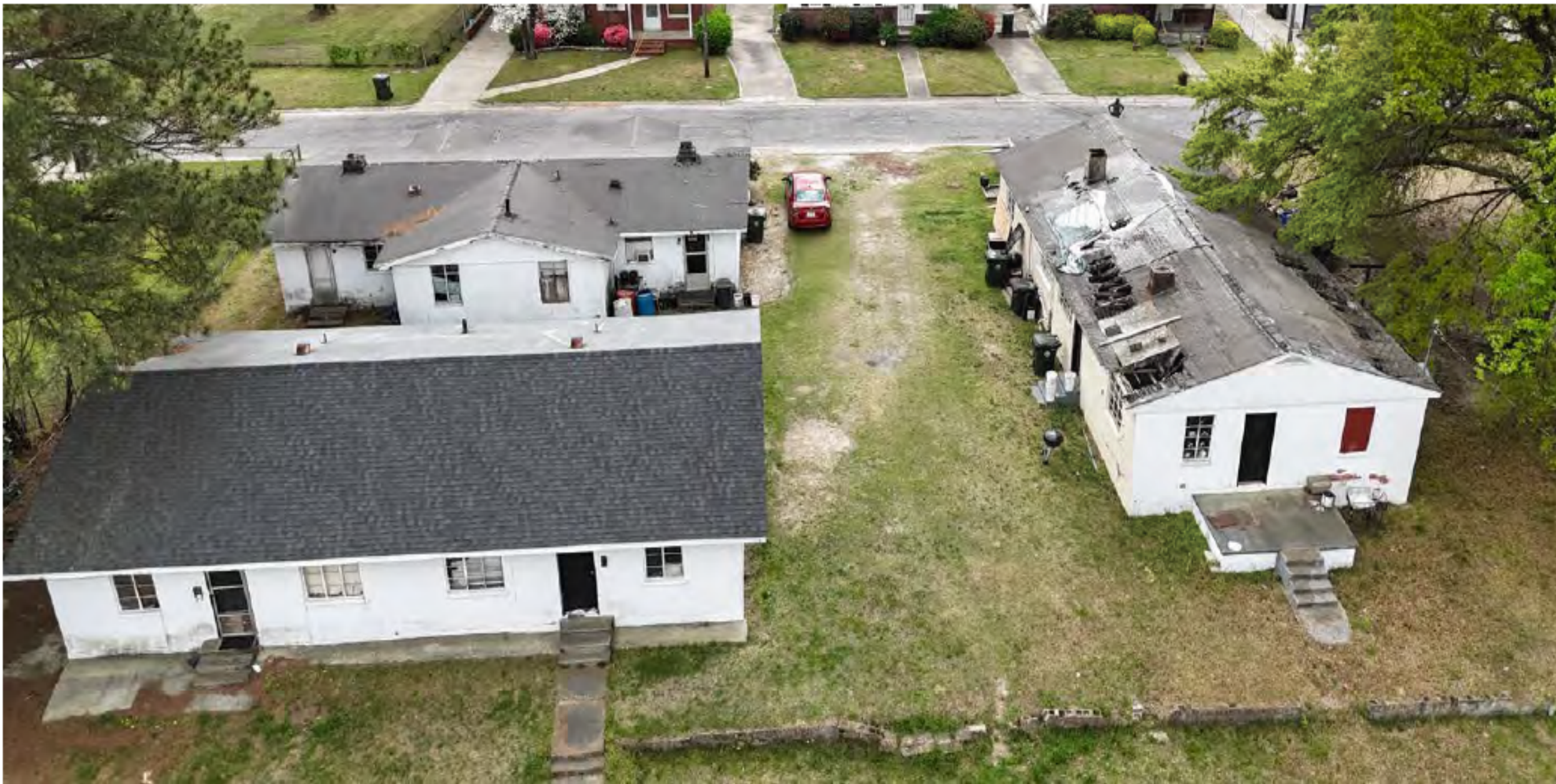
Aerial of Existing Building Conditions @ Olivia Lane
