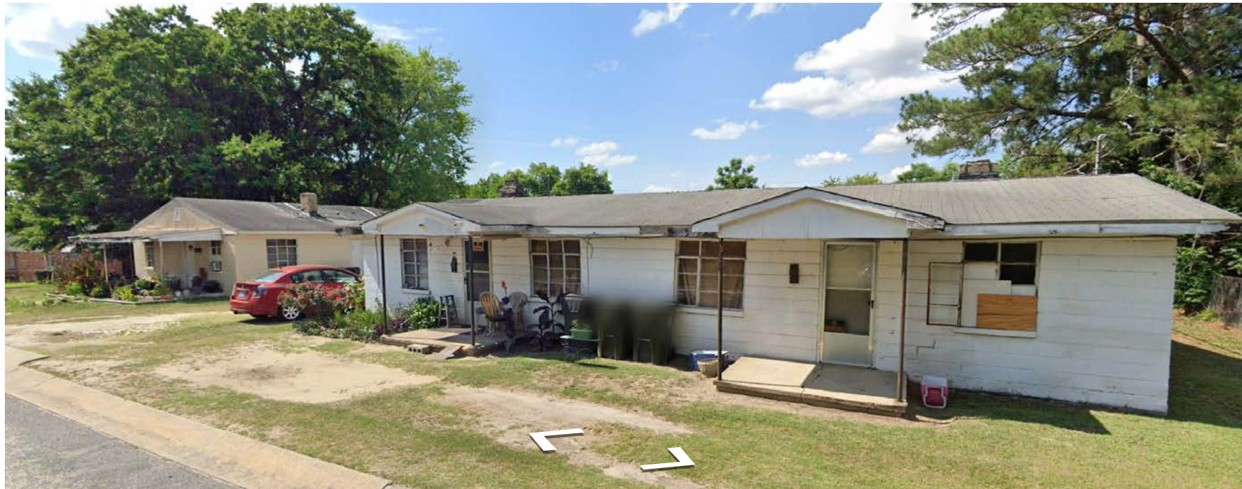
313/315 Existing Building Conditions @ Wilmington Ave
