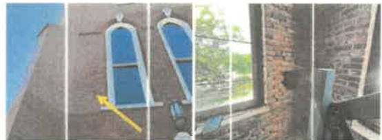
Newer Exterior Pressed Brick Location
