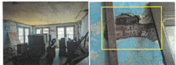
Second Floor storage room
