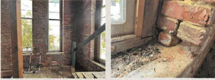
NORTHWEST TOWER (CORNER OF E. CHESTNUT & S. JOHN)
