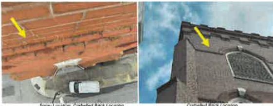
Spray Location, Corbelled Brick Location
