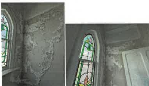
Damaged Plaster/Paint
