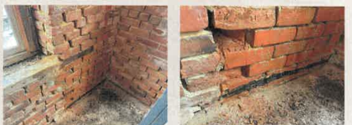
NORTHWEST TOWER (CORNER OF E. CHESTNUT & S. JOHN)
