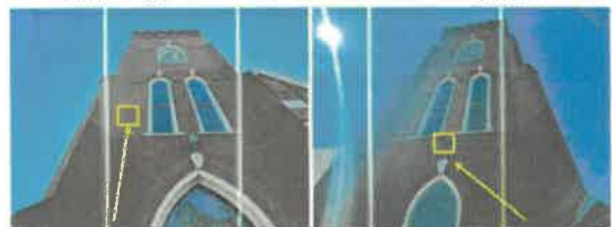
Excavation #02 - Approximate Location of Interior of Excavations North Tower – Excavation #03
