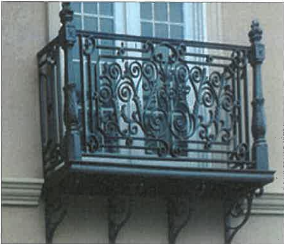
Top and above: Examples of Juliet balconies.
